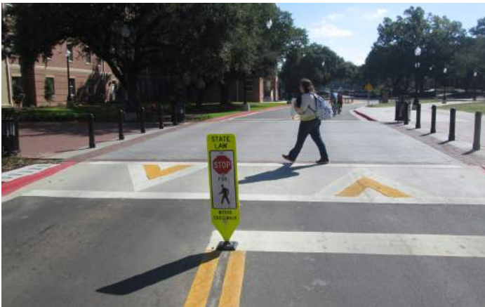
Raised crosswalk on the USM campus prioritizes pedestrian travel.
