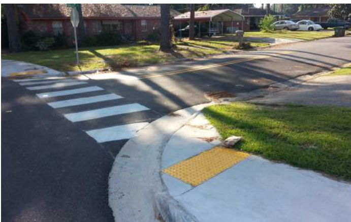
ADA ramps and high visibility crosswalks improve the visibility of pedestrians and help all ages and abilities cross streets.
