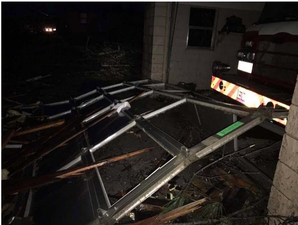
Figure 4. South east face — Bay doors blown in, windows blown in, fire engine damaged
