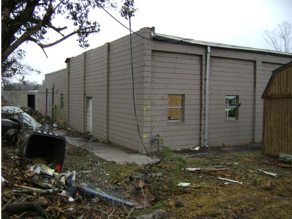
Figure 13. Damaged gutter and downspouts, damaged parapets, flashings and counter flashings. Damaged windows. Damaged gas service.
