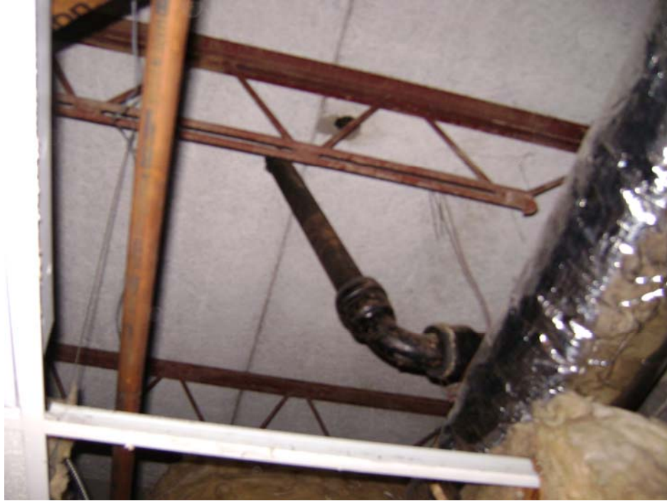
Figure 19. Typical plumbing stack damage multiple locations
