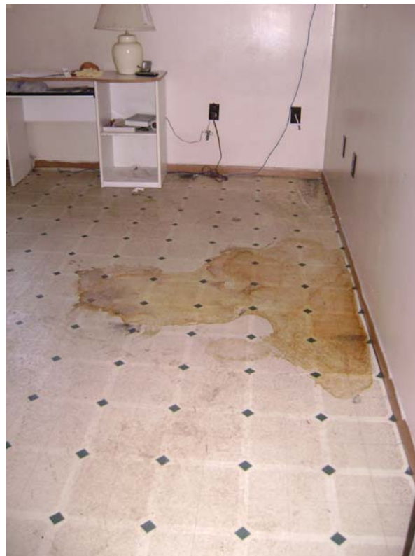
Figure 19. Typical plumbing stack damage multiple locations
