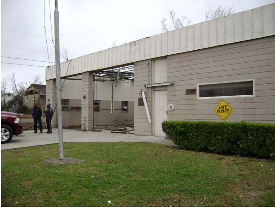
Figure 7. East elevation— canopy loss, door/window damage, wall damage, HVAC damage, glazing damage, fascia damage, flagpole damage
