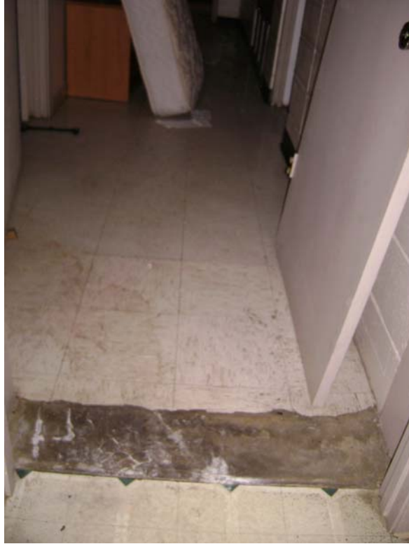
Figure 21. ACM flooring requiring testing/abatement
