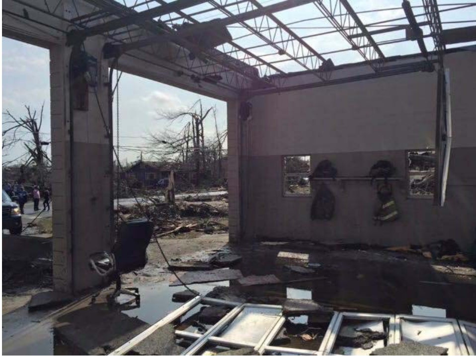
Figure 3. South east face — Bay doors blown in, Roof deck lifted, windows blown in
