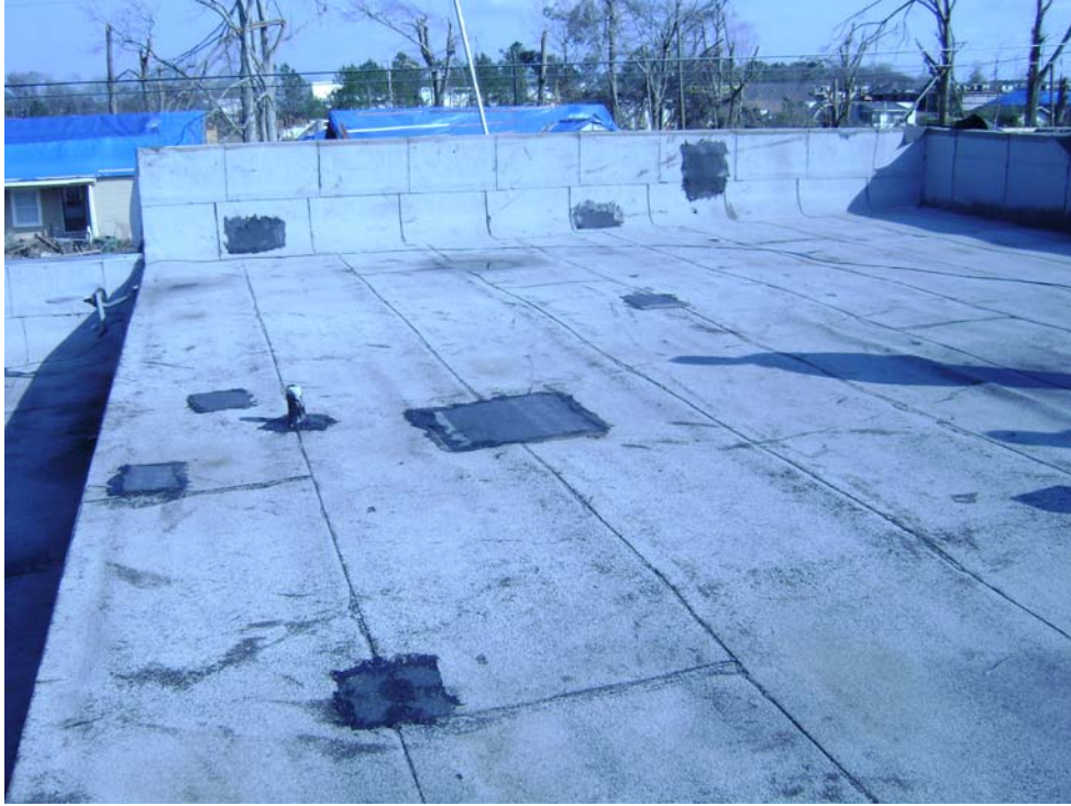
Figure 17. Lower roof damage multiple locations
