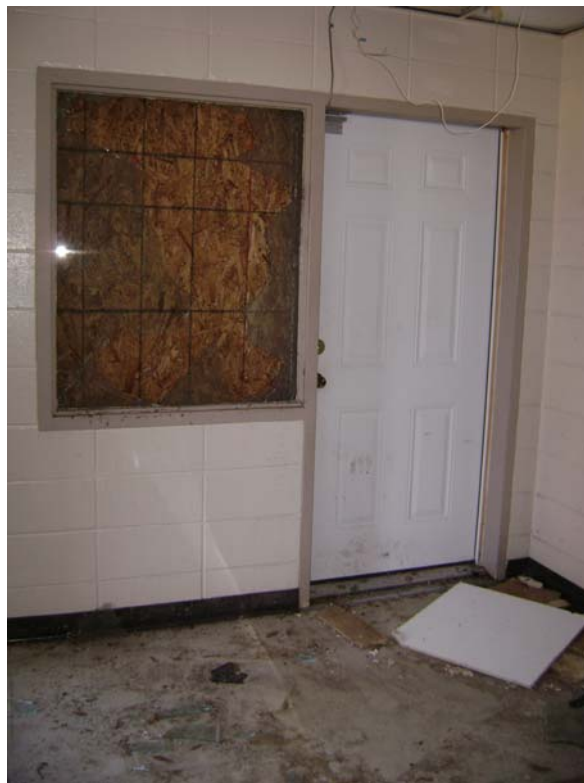
Figure 28. Non fire rated windows breached during storm event
