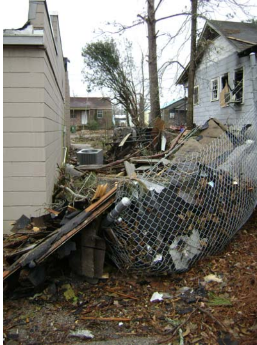
Figure 11. Site— new exterior surrounding 6'-0" cyclone fence with apparatus vehicle gate total loss
