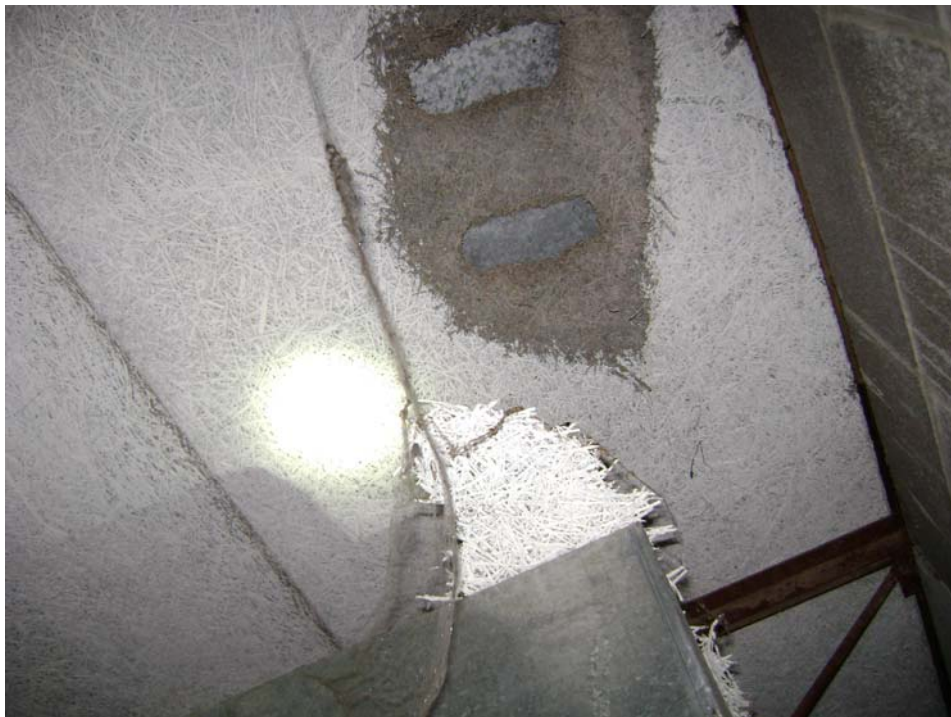
Figure 14. Typical roof decking puncture, wet and damaged roof decking, ceiling, mold infestation, damaged electrical and HVAC
