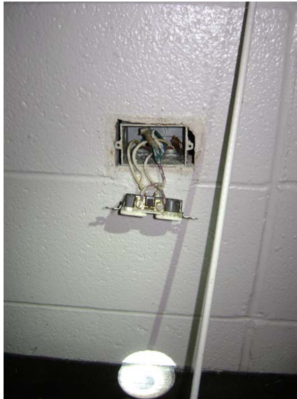
Figure 22. Two wire electrical service all locations
