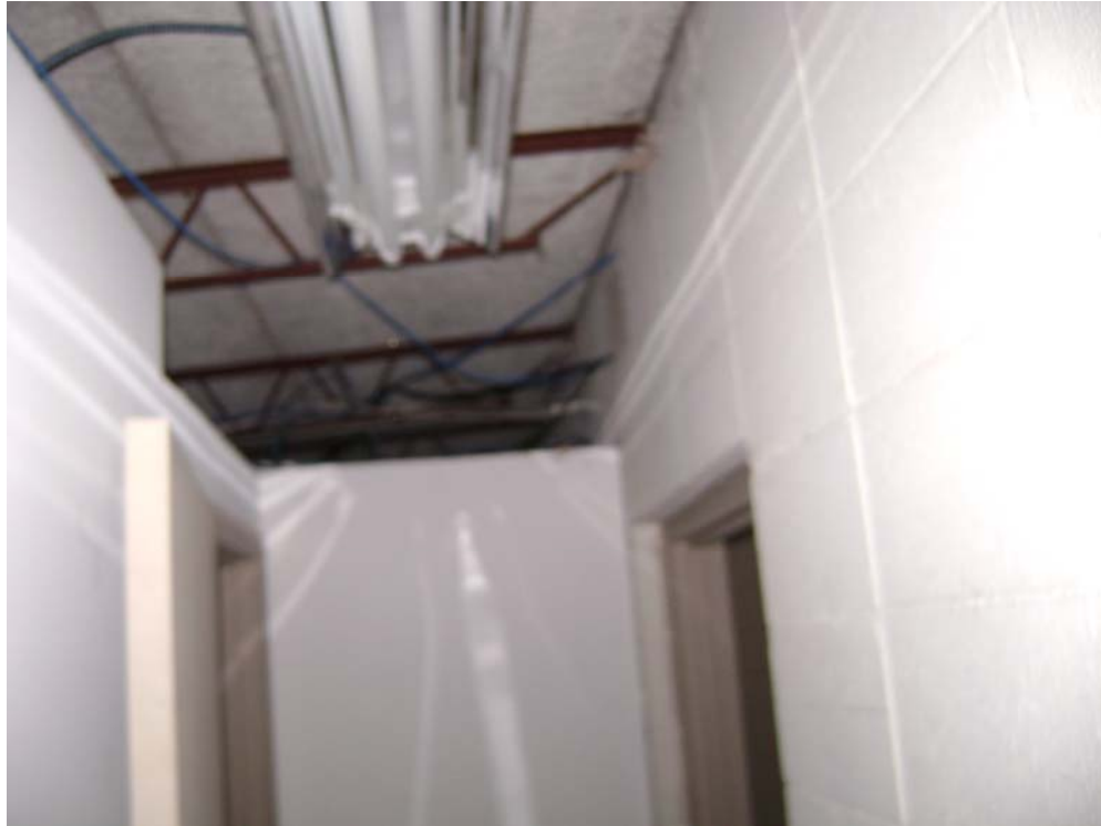
Figure 27. Corridor ceiling stops below roof deck, non-code compliant
