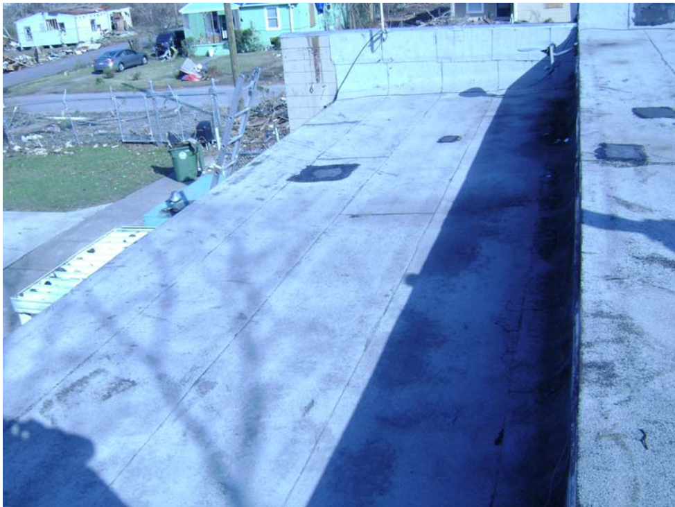
Figure 18. Multiple antennae loss, multiple lower roof penetrations
