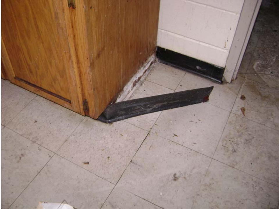
Figure 23. Wet and molding woodwork
