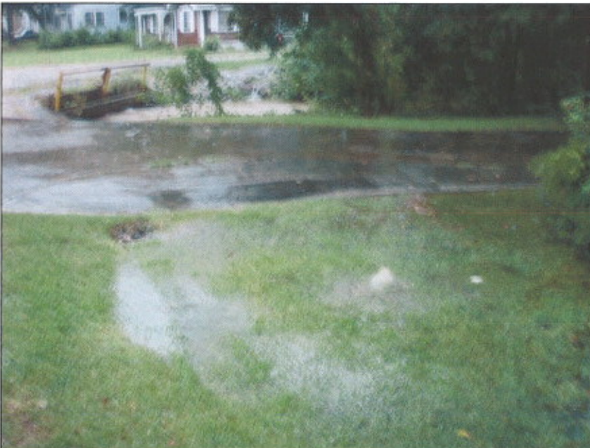
Figure 7. Stormwater canal at N. 19 th and Pearl St. The arrow is pointing at a visible SSO emanating from a lateral within the City's right of way at 200 N. 19 th Avenue in the resident's front yard (See Figure 8.)
