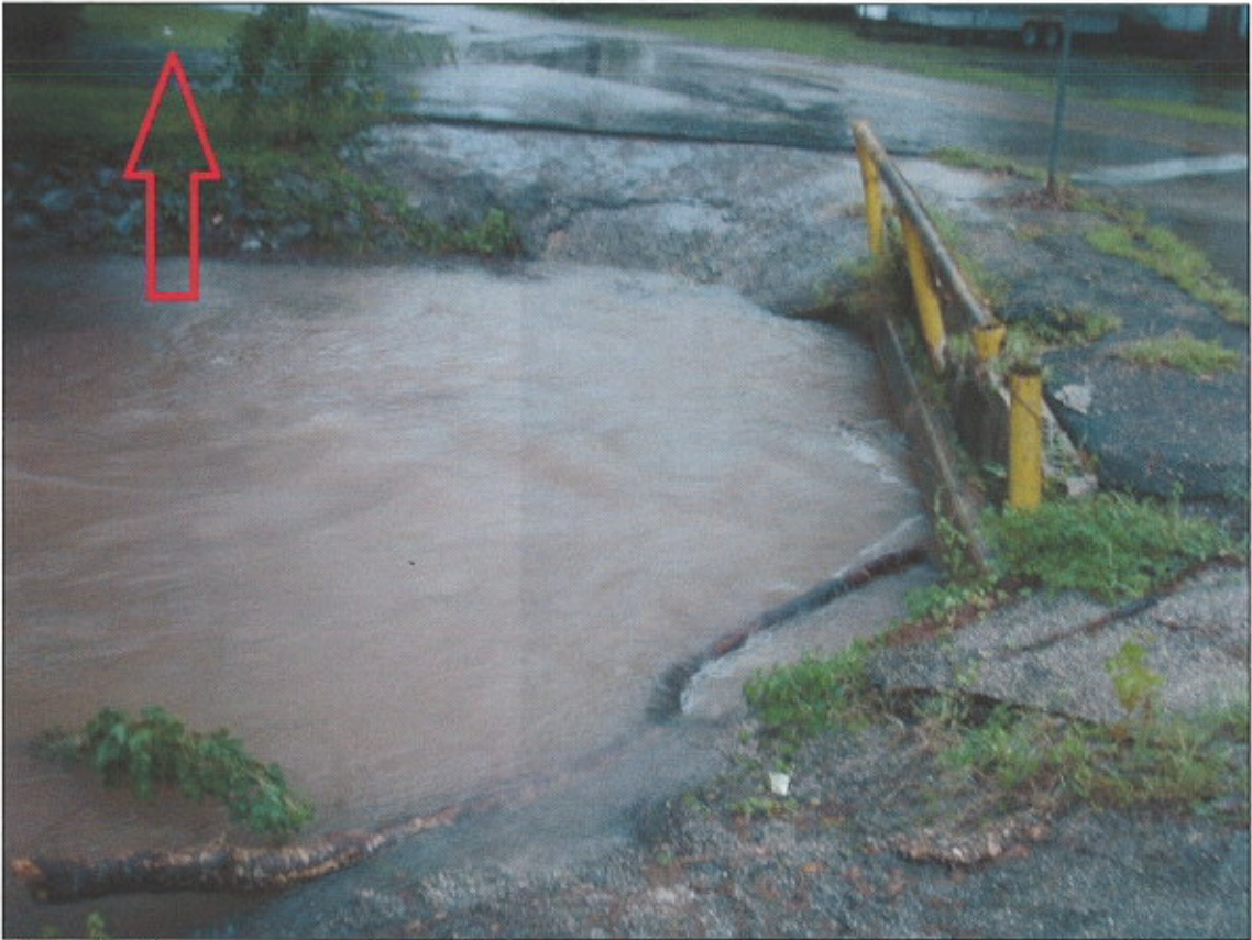
Figure 7. Stormwater canal at N. 19 th and Pearl St. The arrow is pointing at a visible SSO emanating from a lateral within the City's right of way at 200 N. 19 th Avenue in the resident's front yard (See Figure 8.)
