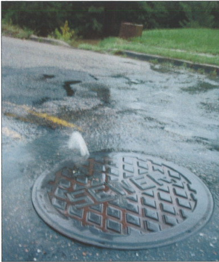
Figure 11. SSO at 105 Park Avenue. Sewage was being discharged into the stormwater canal in the background.
