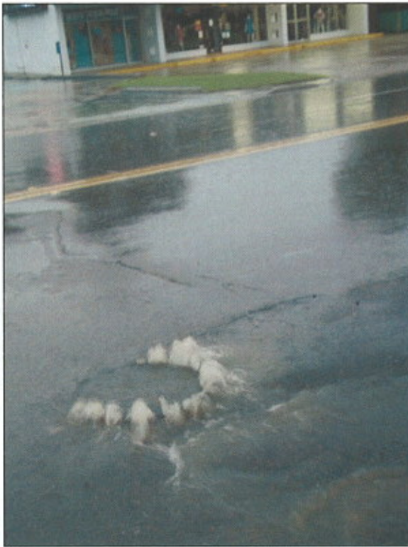
Figure 6. SSO on Hardy Street in front of the Sunflower Grocery Store. Note the indentation of the asphalt on one side of the manhole cover, indicative of chronic surcharging.
