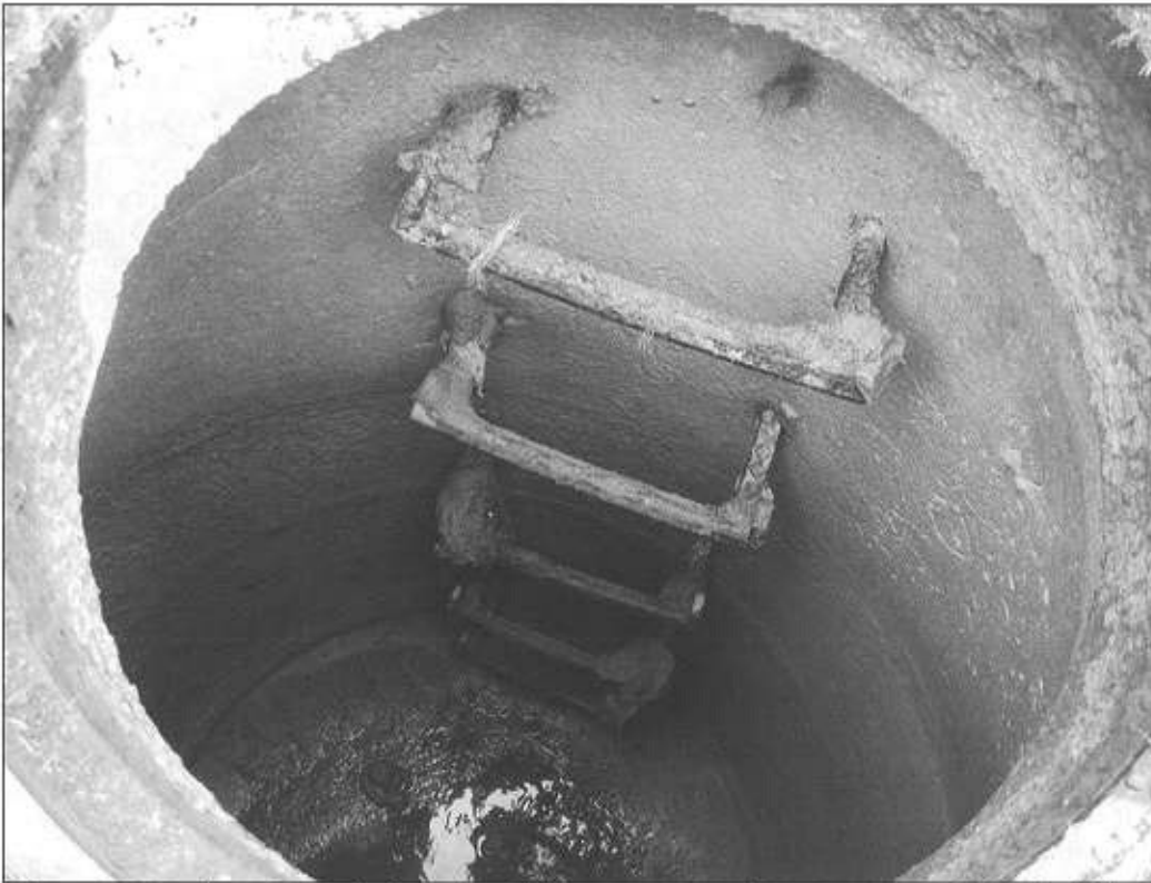
Figure 5. Interior of manhole at N. 19 th Ave and Pearl Street. Note debris build-up on the top ladder rung as well as the lower elevated ladder rungs.
