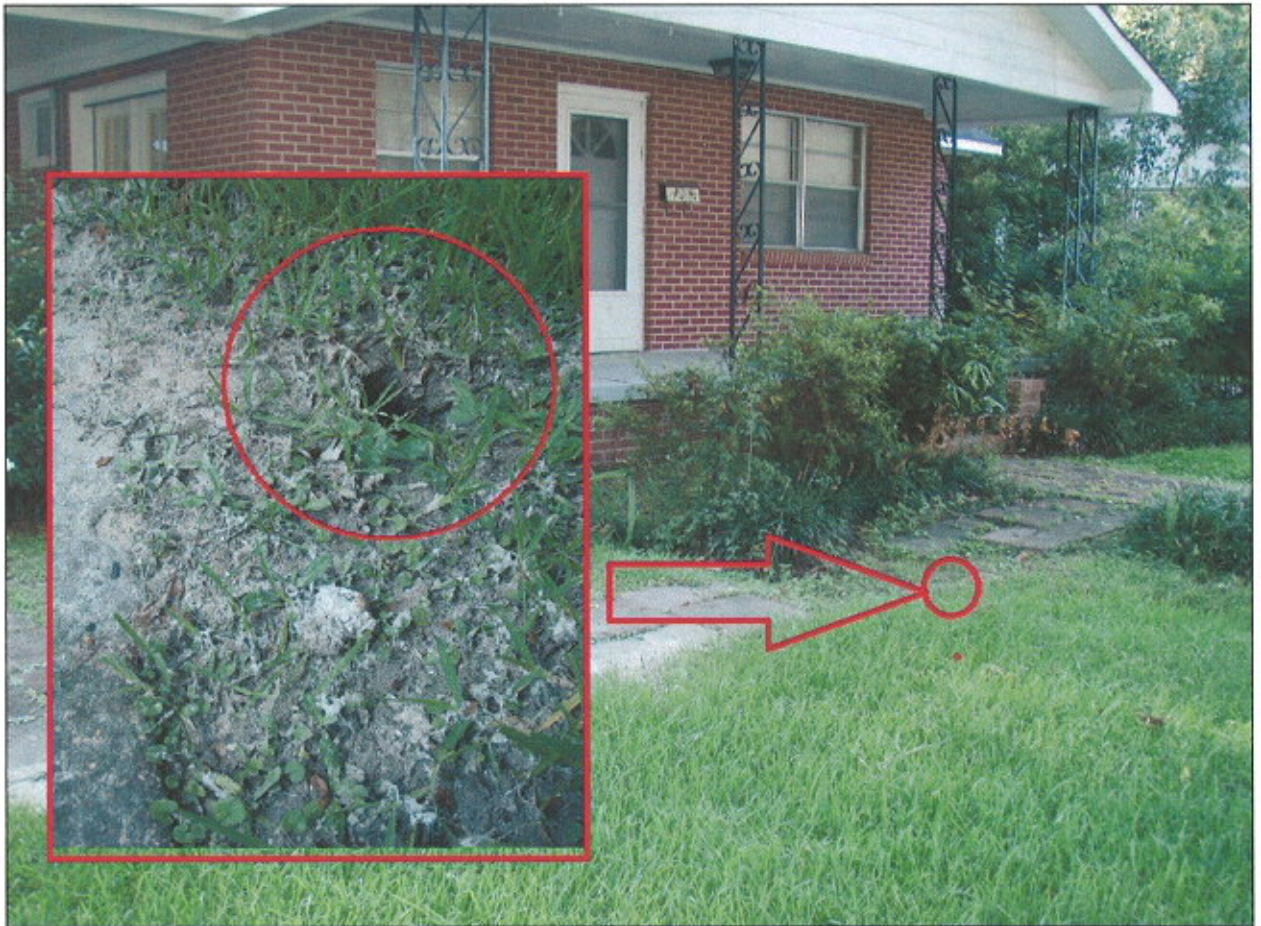
Figure 4. The arrow shows the location of a 3 to 4 inch diameter hole surrounded by sewage debris located in residential yard.
