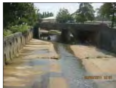
Ronie Street Creek View of Crossing
