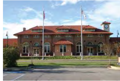
27 Newly restored Hattiesburg Train Depot
