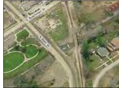
Bird's Eye View of Crossing
