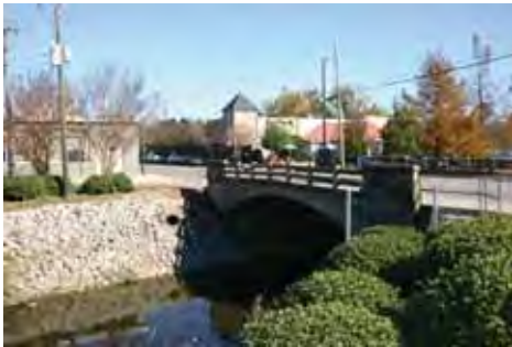
Concrete bridge over creek on Walnut Street
