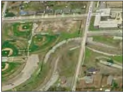
Bird's Eye View of Crossing
