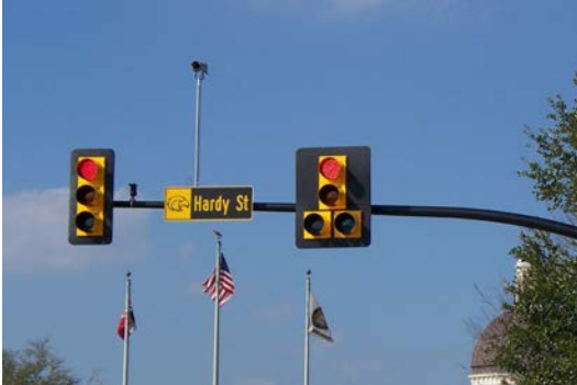
Photo: New mast-arm traffic signal on Hardy Street at the entrance to the University of Southern Mississippi.
