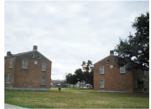
Briarfield Homes Apartments, built in 1941 with the assistance of the U.S. Department of Housing and Urban Development
