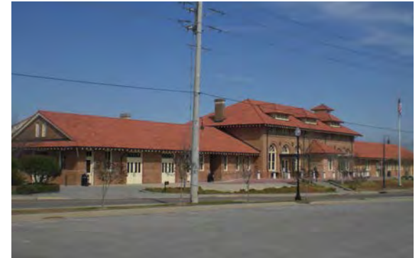
Recently Restored Hattiesburg Depot, built in 1910 in the Italian Renaissance style
