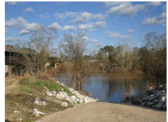
Boat Access to Leaf River at Old Highway 42 Bridge
