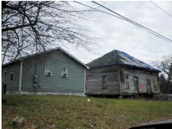
An occupied home adjacent to a home in disrepair
