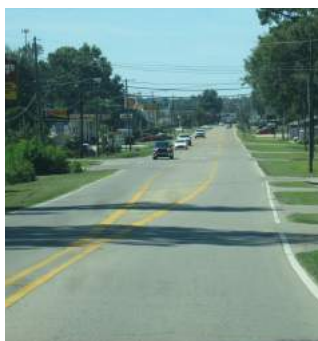
Central Avenue in Petal lacks sidewalks on both sides of the main street .
