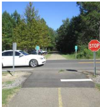
Approaches to trail crossings along roadways lack signage and/or pavement markings to alert motorists about trail crossings.
