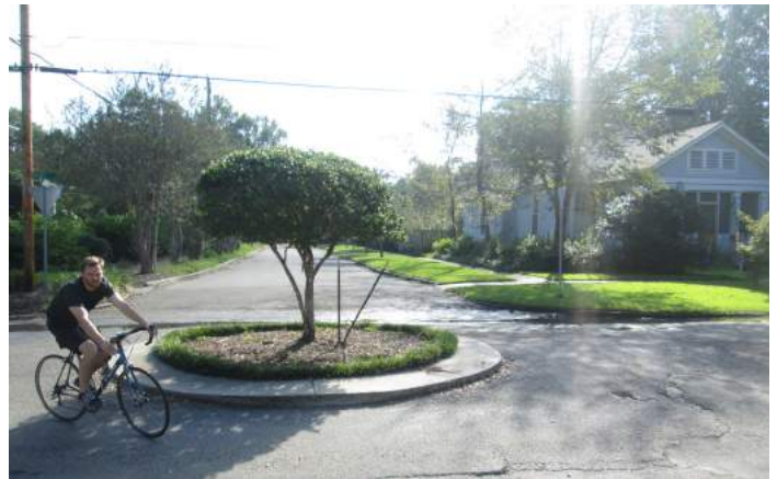
Traffic circles result in calm neighborhood streets by slowing vehicles through intersections.
