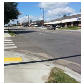
Major intersections lack dedicated space for bicyclists to cross comfortably.
