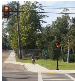
Some sections of trail are narrow and do not provide adequate buffers between the path and the roadway.
